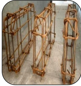
Figure 5: Conventional Steel Cage
